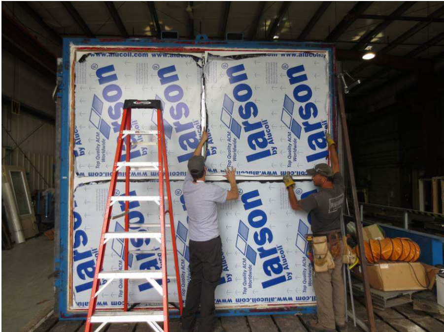
Figure B3 – Upper Panel Installation
